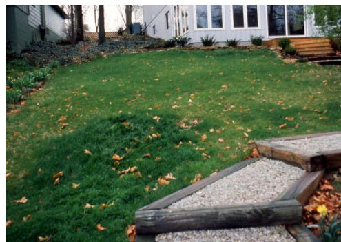
Grass over the septic tank should NOT be green
