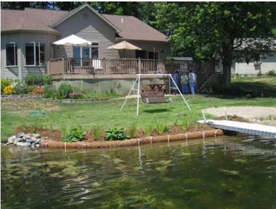
Figure 7. Seawall after shoreline stabilization using bioengineering techniques.
