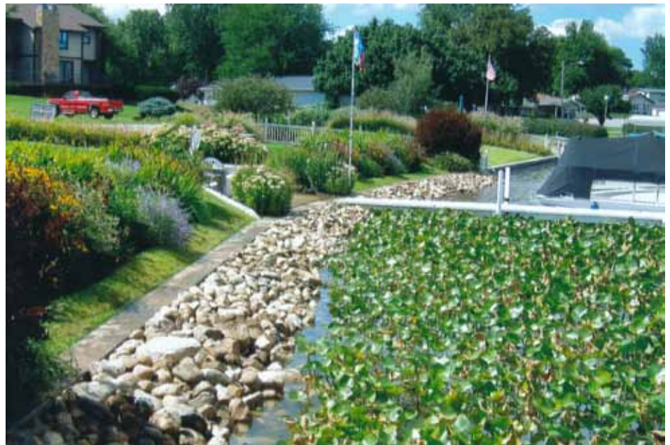
Figure 5. Seawall after new glacial stone improvements.
