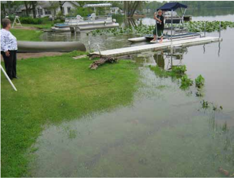
Figure 6. Seawall, prior to shoreline stabilization using bioengineering techniques.
