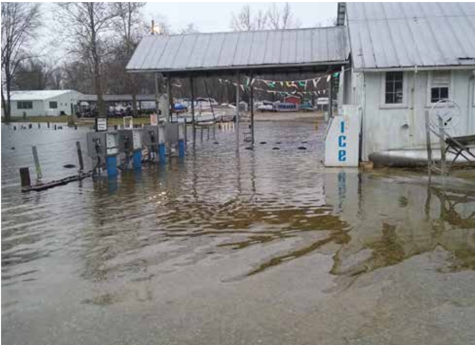
Figure 11. Gas station in Patona Bay, taken 2/25/18.
