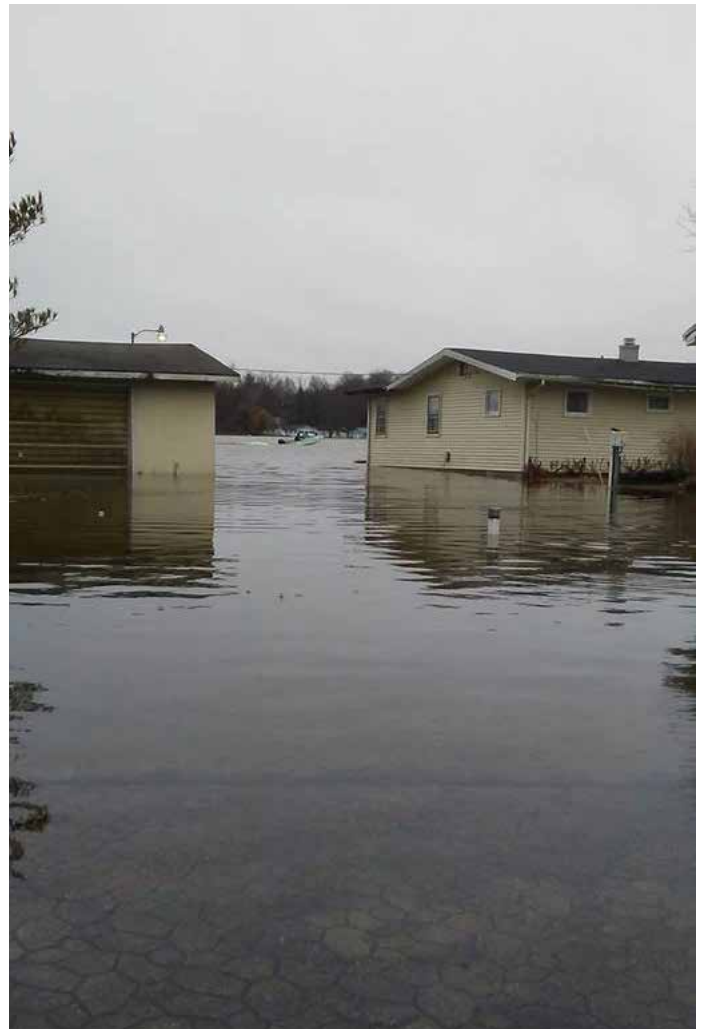
Figure 10. Flooded houses on Barbee Chain. Photo by John Labriola.
