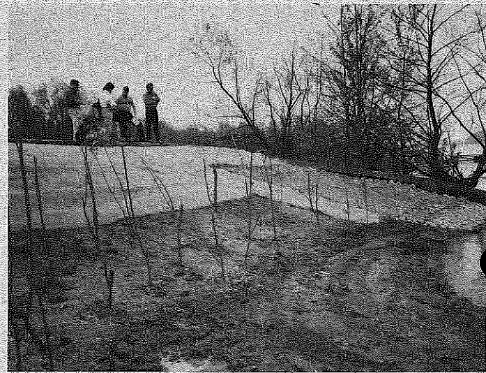
Conference participants view shoreline erosion control demonstration site at the Paynetown boat ramp. Measures pictured are: willow posts (foreground), articulated blocks (right background), and erosion control blanket on seeded area (left background).
